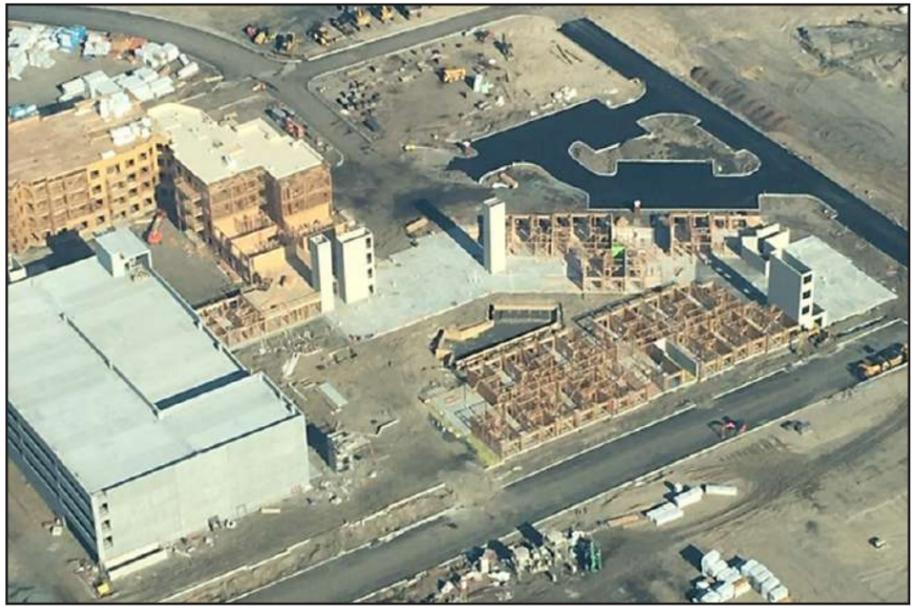
An aerial view of the Manhattan Beach Project at South Amboy waterfront shows the completed parking deck, elevator shafts and roof membranes currently being constructed. South Amboy on the move! (Photo/info courtesy of Jorge Gonzalez-Gomez)
