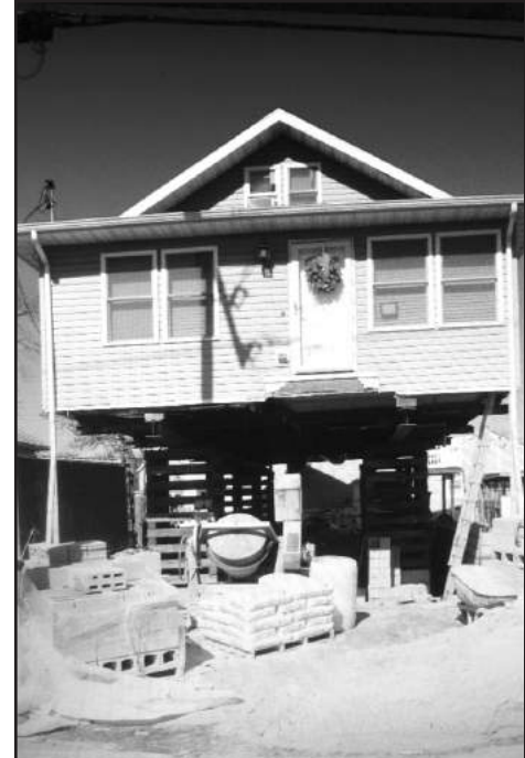
This house located at 104 Henry St., South Amboy, was the home of the late Stanley Ziobro. The structure was badly damaged by Superstorm Sandy in 2012, and is finally seeing some improvements being done. Owner Mary Lou Ziobro Mickiewicz said, "After the dilemma of my being misplaced by a private contractor, work is at last being done, and the house is finally being elevated. My son Robert Mickiewicz and his wife Ashley came all the way from South Dakota to help me." (Photo by Tom Burkard)
