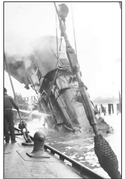
May 15, 1943-This engine went off the end of the Powder Pier in South Amboy into the Raritan Bay, and is pictured being raised out by Merritt & Chapman Crane, which was working in New York at the time. (Photo/info courtesy of George Selover)
