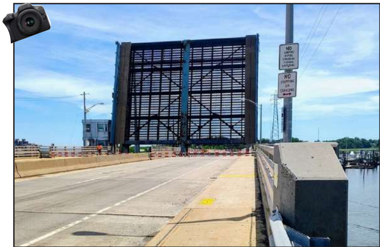
Morgan Bridge (Rt 35) Spans the Cheesequake Creek between the Morgan section of Sayreville and Laurence Harbor
