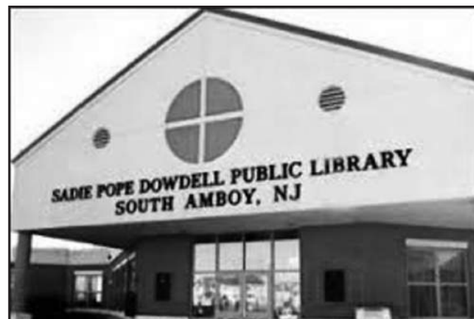
Dowdell Library's current location at HG Hoffman Plaza, South Amboy.
