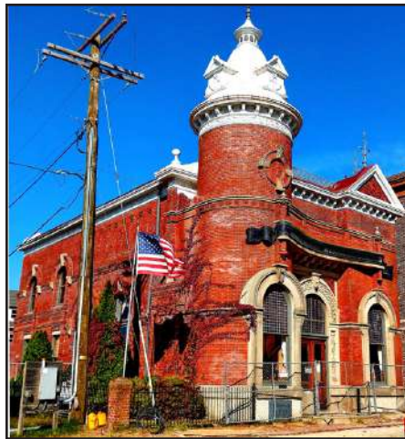
November-Where in New Jersey Salem Municipal Building, Salem New Jersey
