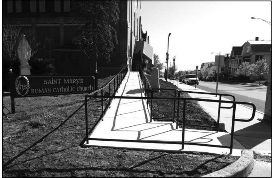
The new handicap ramp at St. Mary's Church has been completed, and is ready for use by the parishioners who require it. (Photo/info by Joe Lotkowitz)
