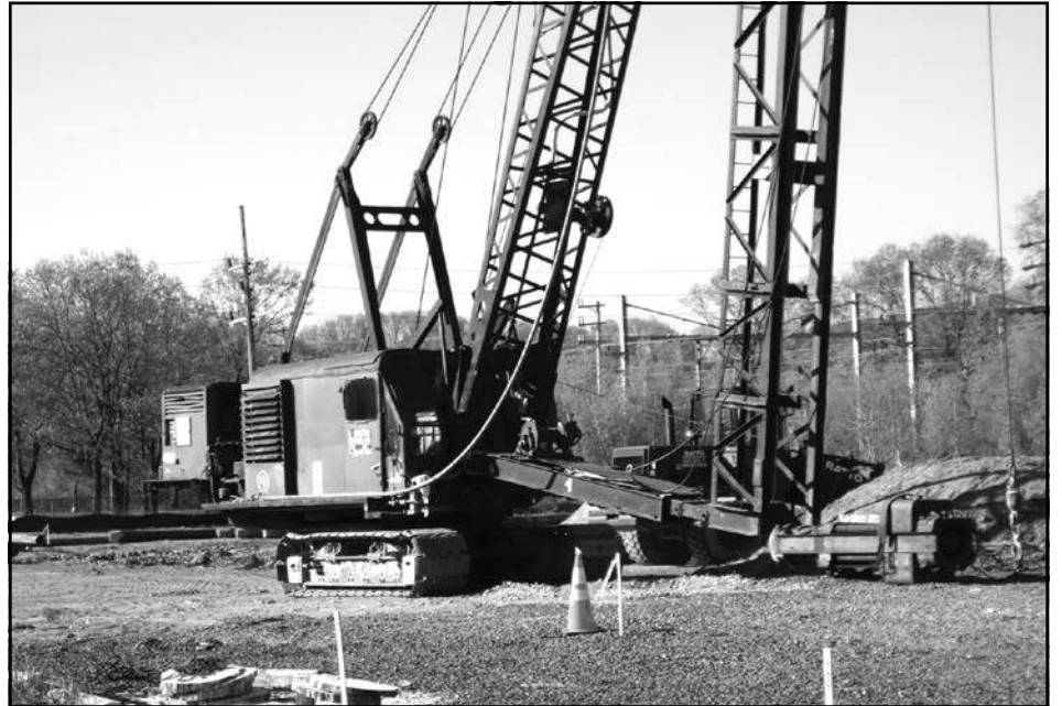
New Townhouses -Construction at Bay Side of South Amboy Luxury Townhouses at the entrance of Waterfront Park has begun. The heavy equipment pictured, is putting in the pilings that will anchor and stabilize the base for the footings of the townhouses that will be constructed, when all the preliminary rough work is completed. The time table for occupancy has not yet been determined. The townhouses will conform with FEMA construction regulations and guidelines as required after Superstorm Sandy. (Photo/story by Joe Lotkowitz)
