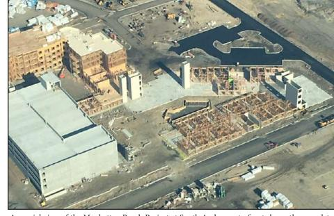
An aerial view of the Manhattan Beach Project at South Amboy waterfront shows the completed parking deck, elevator shafts and roof membranes currently being constructed. South Amboy on the move! (Photo/info courtesy of Jorge Gonzalez-Gomez)
