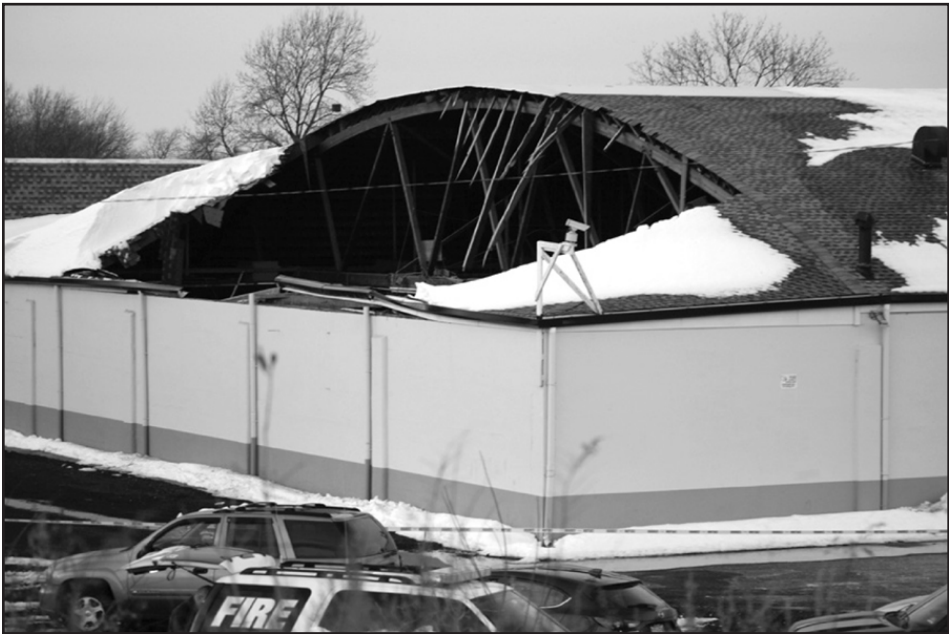
On January 26, 2016 the back roof of the RollerMagic Skating Rink in South Amboy collapsed from a large amount of snow that was piled up on a section of the roof. Local emergency services turned in an exemplary job of responding to the call, and all gas and electricity was turned off as a precautionary measure. Upon getting access to the interior of the building, officials reported many broken support beams that were deteriorating, according to reports. Fortunately no one was injured at the time of the collapse. (Photos by Tom Burkard)
